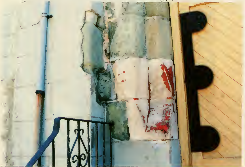
North Elevation of Church Building (M)
